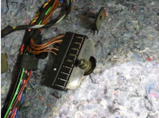
Factory Grounding Point
