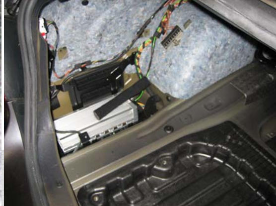
Photo for reference of Ground Location
